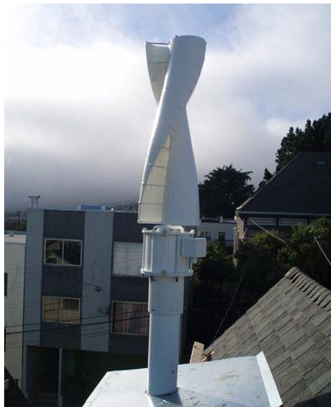
Vertical Axis Wind Turbine
